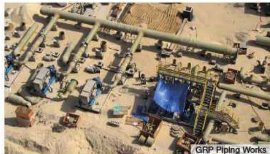
GRP Piping Works
